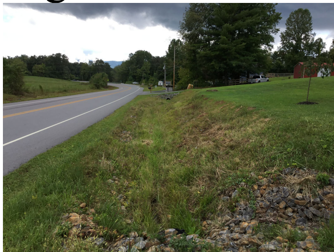
Site 4 Photo Point #2 (Downstream)
